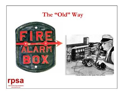
It was not uncommon in the early 20th century to have initiating devices (thermostats, sprinkler waterflow switches and manual boxes) connected to a circuit that directly controlled bells connected in the fire house. One property, one bell. In another configuration, an automatic coded telegraph transmitter might be used on a city or privately owned telegraph circuit.
