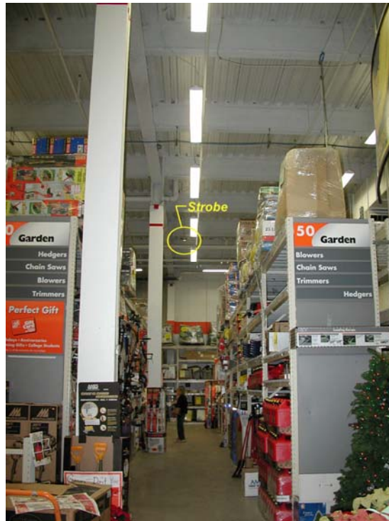
Photo 1 - Strobe Over Aisle (Reading, MA)
